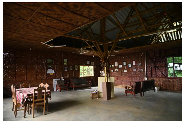
North East Network's Resource Centre, which has been designed and built with local materials.
