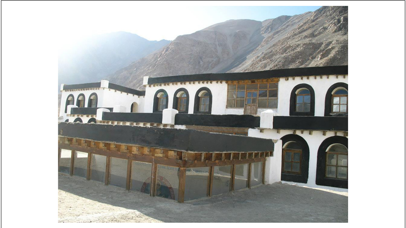
Figure 2. Changthang school, an example of a solar-earth building created locally in Ladakh (Source: N. Joshi).
