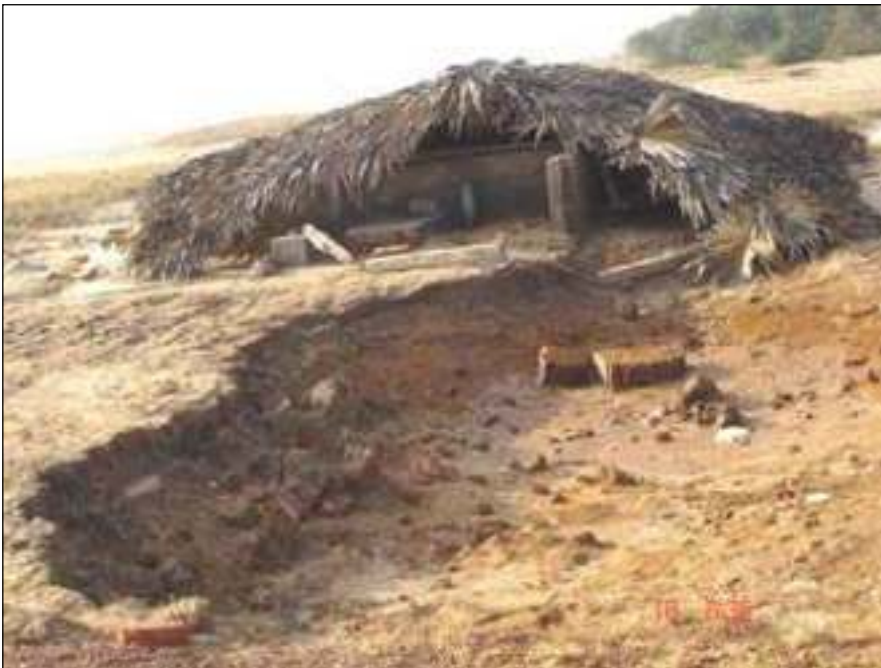
Figure 15. Mud house with thatch roof built within 100 meters of the sea at Pakala Beach in Andhra Pradesh (photo: Arvind Jaiswal).
