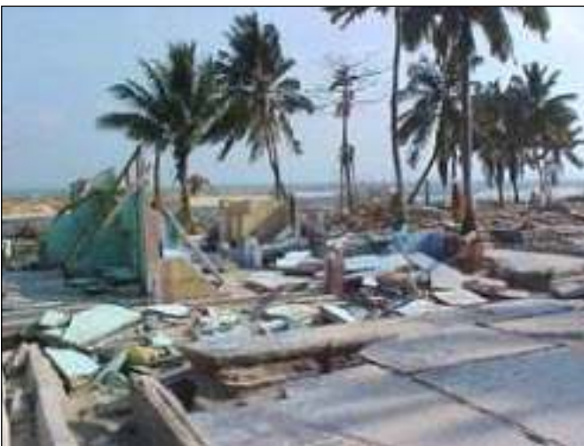
Figure 6. General destruction of built environment at Hut Bay in Little Andaman Island (photo: C.V.R. Murty).
