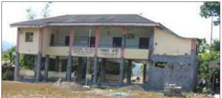
Figure 9a. The Panchayat Bhavan building showed severe cracking and damage to the soft first-story columns and infill walls (photo: Durgesh C. Rai).
