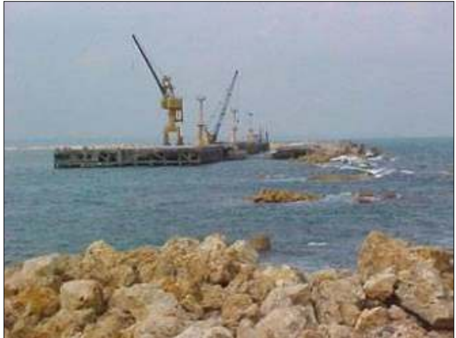
Figure 11. Shortage of appropriate construction material forced the use of porous coral stones from local quarries for building the breakwaters. The stones were easily uplifted during the tsunami and breached a large segment of the approach to the RC jetty at Hut Bay (photo: C.V.R Murty).
