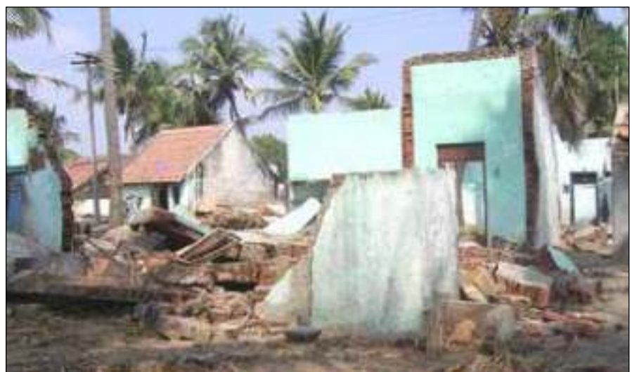
Figure 14. Houses destroyed by the waves at Nagapattinam in Tamil Nadu (photo: Alpa R. Sheth).
