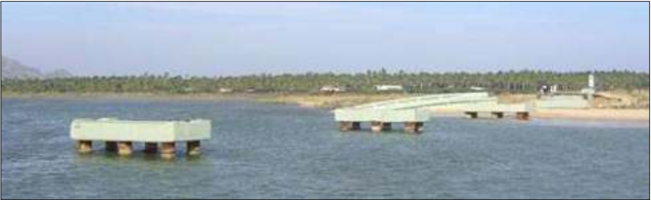
Figure 17. Complete loss of spans of the four span RC bridge at Melmannakudi in Tamil Nadu (photo: Alpa R. Sheth).
