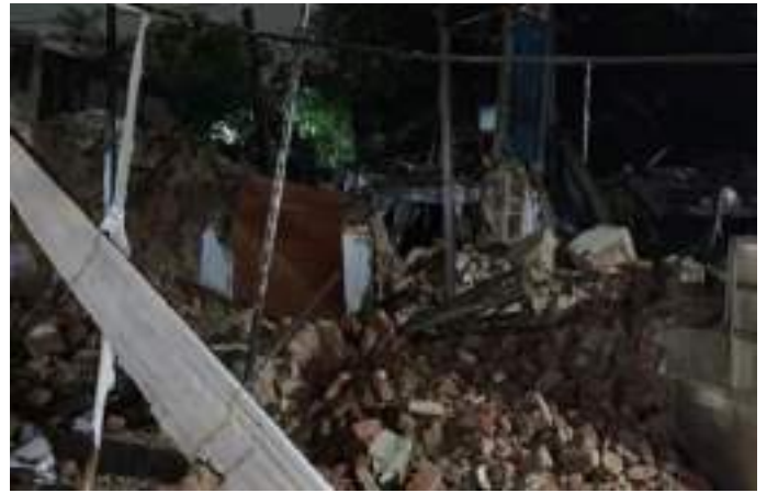
Hyderabad Floods: Downpour claims 40 lives in rain-related incidents in five days
