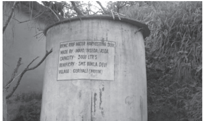
A roof water harvesting tank [image by: WAFD]
